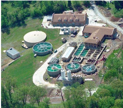
Aerial view of a water treatment plant.
